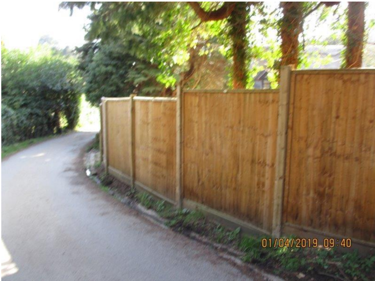
Figure 5 – Photo of fencing after gates
