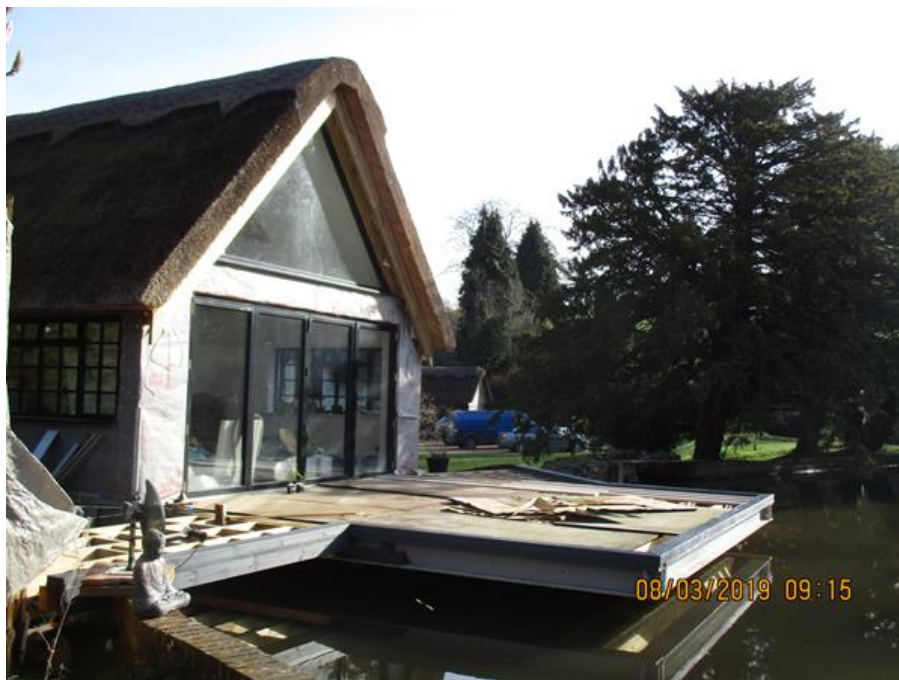
Figure 3 – Photo taken by the Case Officer on the site visit showing the rear extension and decking
